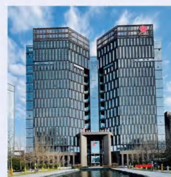
Construction service center in Hangzhou
