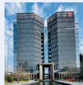
Construction service center in Hangzhou
