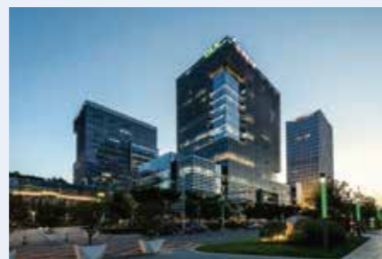
R&D and sales center in Nanjing
